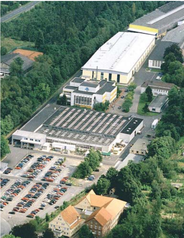
Piller Headquarters & Manufacturing Facility, Osterode
